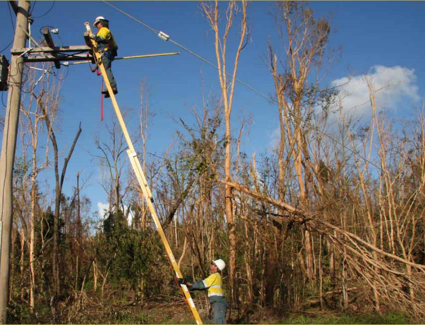
Ergon Energy workers restore power in Far North Queensland after Cyclone Yasi. © The State of Queensland.
