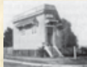
National Bank of Australasia moves into a new timber triangular building known locally as the 'Wedge of Cheese'.
