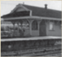
Electricity is installed at the railway station.
