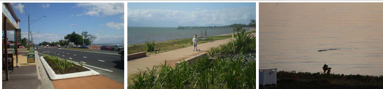
Above: Reconstructing Cardwell completed works, September 2013—roadway (left) and common use pathway (centre) - and locally known Cyril the Croc who kept a watchful eye on works (right)
