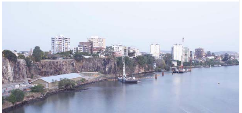
Above: a view of the works underway from the Storey Bridge.
