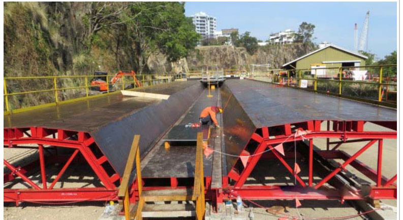
Above: assembly of pre-cast mold for the concrete girders
