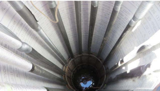
Above: Looking down inside one of piles before the concrete is poured; the steel bars are for reinforcement.
