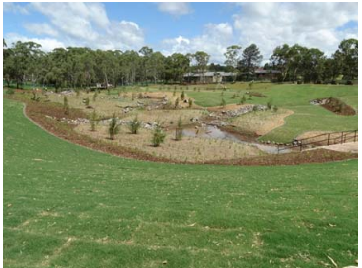
Completed works - Garnet Lehman detention basin
