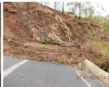
Landslips and damage to the Burnett Highway (Mount Morgan Range) following Tropical Cyclone Oswald (left); and following reconstruction works (right)
